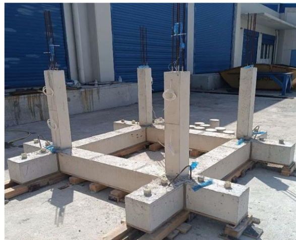
b) Stripping of the foundation and columns
