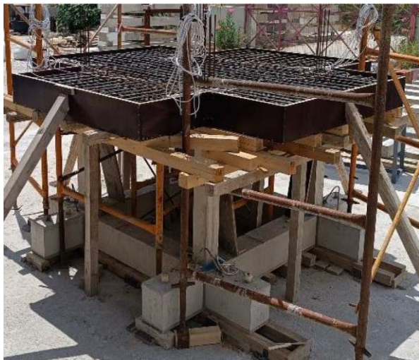
c) Formwork of the slab
